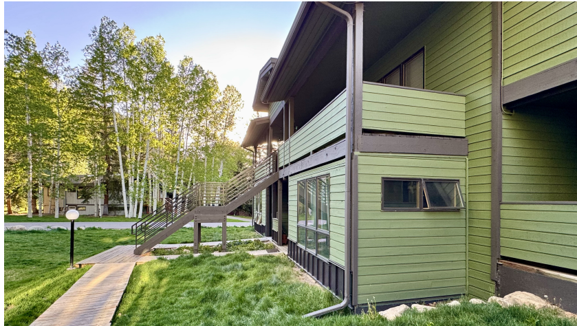
View along the building's side. Walkway access connects the unit's grassy outlook to Cottonwood Rd.
