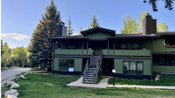
Building H, Par Six Condominiums. Recent exterior repaint and new metal siding.
